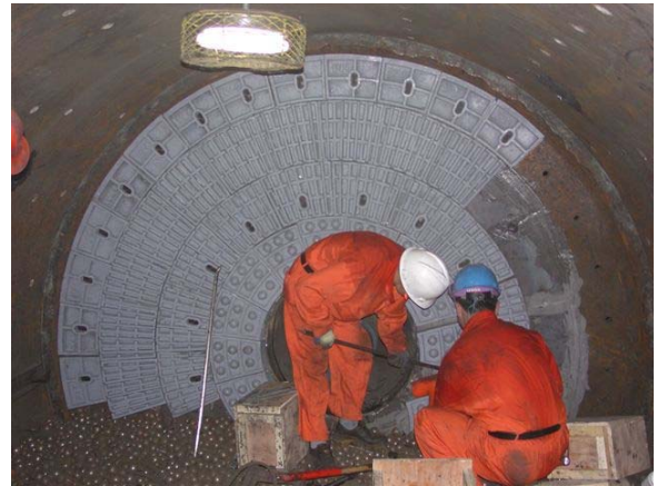
Figure 3. Installation of metal magnetic lining with mill charge in place.
